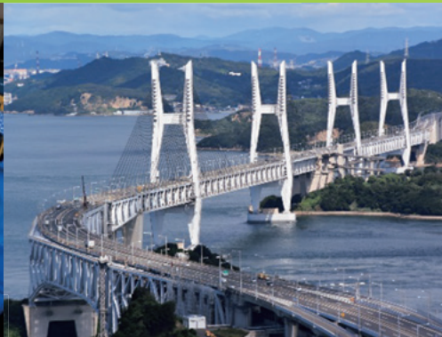
Social infrastructure(Great SetoBridge)
