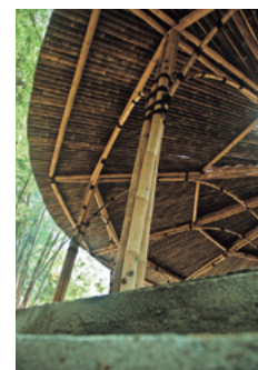
Temporary housing model made of bamboo and plaster in a disaster area of the Central Java Earthquake (Study on reconstruction processes by the Environmental Planning & Design Lab)
