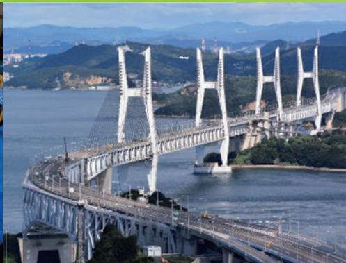
Social infrastructure(Great SetoBridge)
