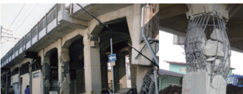
Field surveys on lifeline damages
