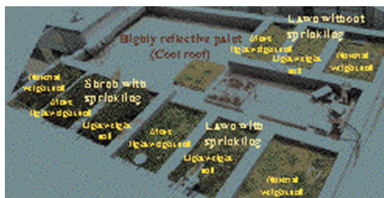
Experimental roof for surface cover technology in an urban structure at Kobe University (Study on urban thermal environment by Assoc. Prof. Takebayashi)
